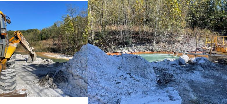
The 309 Discharge is a site of active remediation where the water is being treated to increase the pH and remove iron prior to discharge into the Little Schuylkill River. Following the active treatment, the water flows through a wetland area where iron precipitates prior to entering the Little Schuylkill River.
