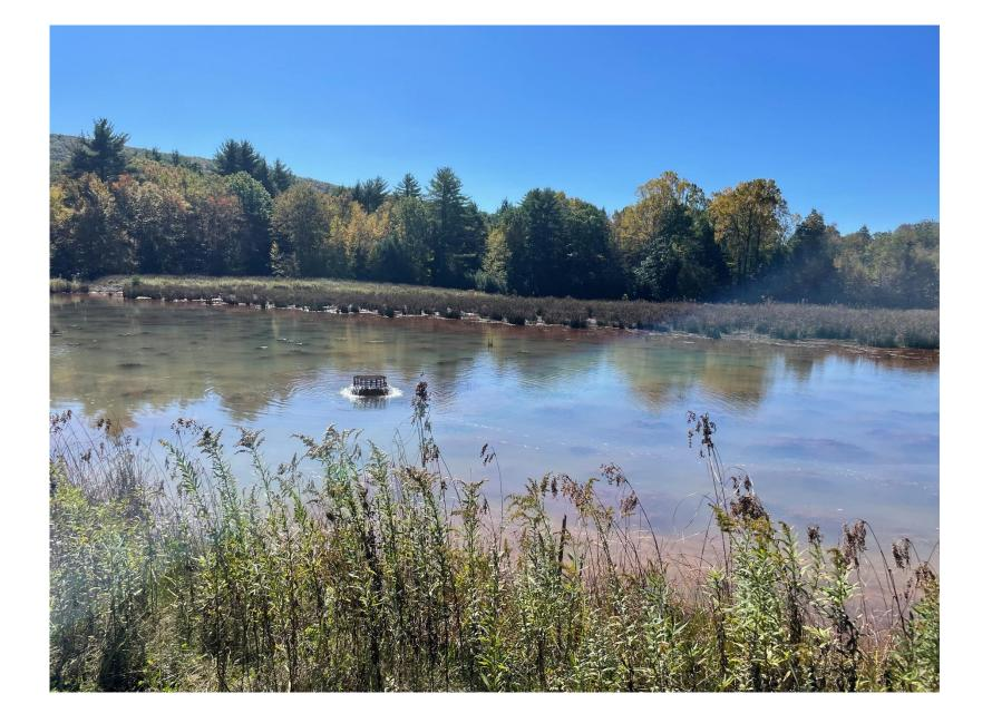
The Schuylkill Conservation District and the Schuylkill Headwaters Association work toward a cleaner watershed through passive remediation projects such as this wetlands at Mary-D. Abandoned Mine Drainage (AMD) enters the system with low pH and high iron levels. The water is passed over limestone to increase the pH. There are a series of pools in which the iron can oxidize and precipitate out of the AMD
